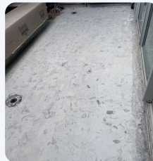
Strip-out to slab
